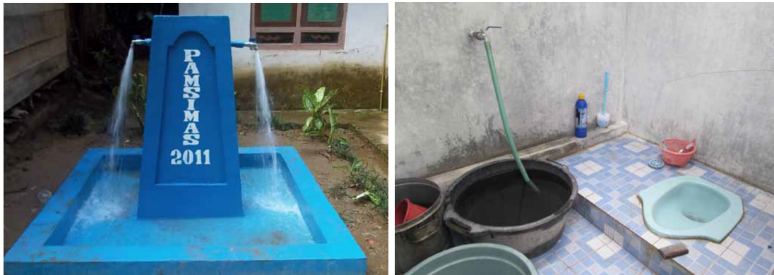
(a) Public Water Tap.
