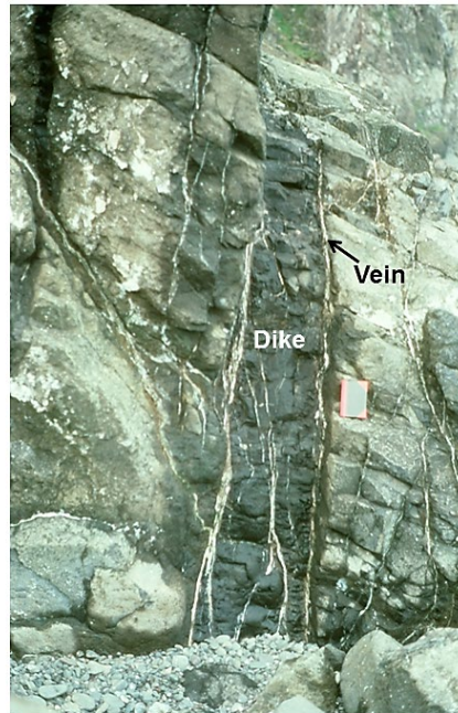
Figure 1. Basaltic dike, providing paths for geothermal fluids, in the damage zone of the Husavik-Flatey Fault, a transform fault partly exposed on land in North Iceland [10,14]. The mineral veins dissect the central part of the dike but occur mainly at the dike contacts with the host rock (one vein is indicated). There stress concentrations encourage fracture formation [17,18], including the propagation of hydrofractures (seen here as mineral veins). View east, the dike is about 0.4 m thick (the height of the red-black notebook at the right margin of the dike is about 15 cm).
