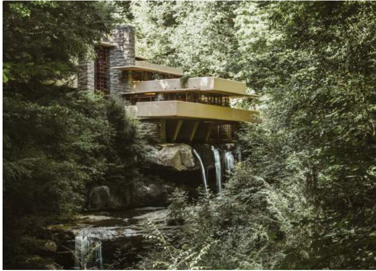
fig. 26 Exemplary cantilevers: Frank Lloyd Wright's Fallingwater, 1935
