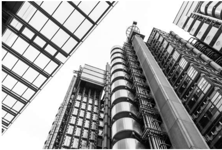
fig. 41 Lloyd's Building, London, 1978
