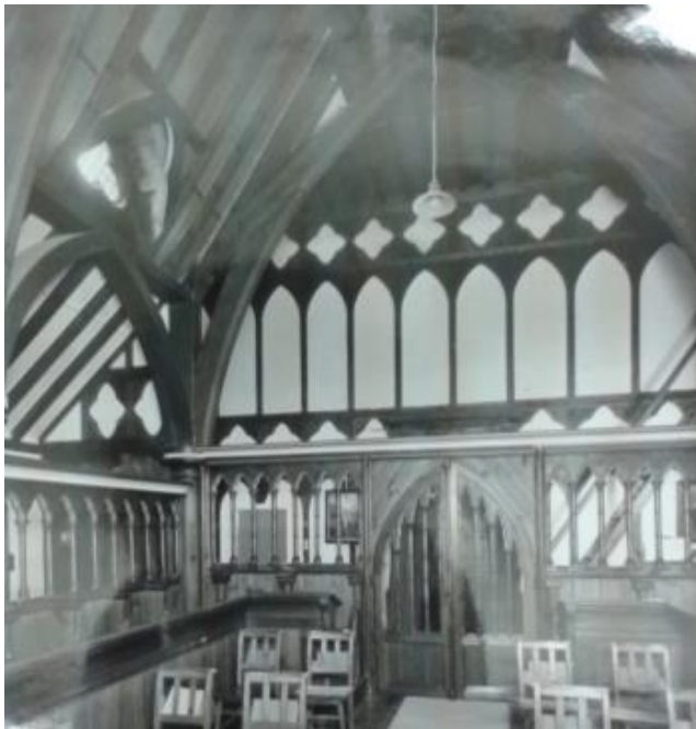
Figure 5.9 Upper room chapel Ditchingham, showing original doors into the choir. Undated.
