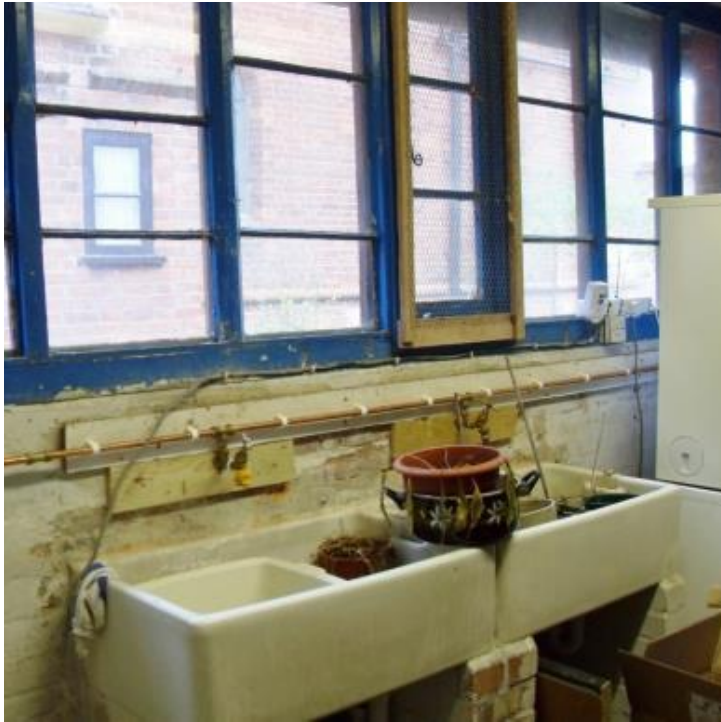
Figure 4.9 Sinks in the original laundry at Ditchingham.
