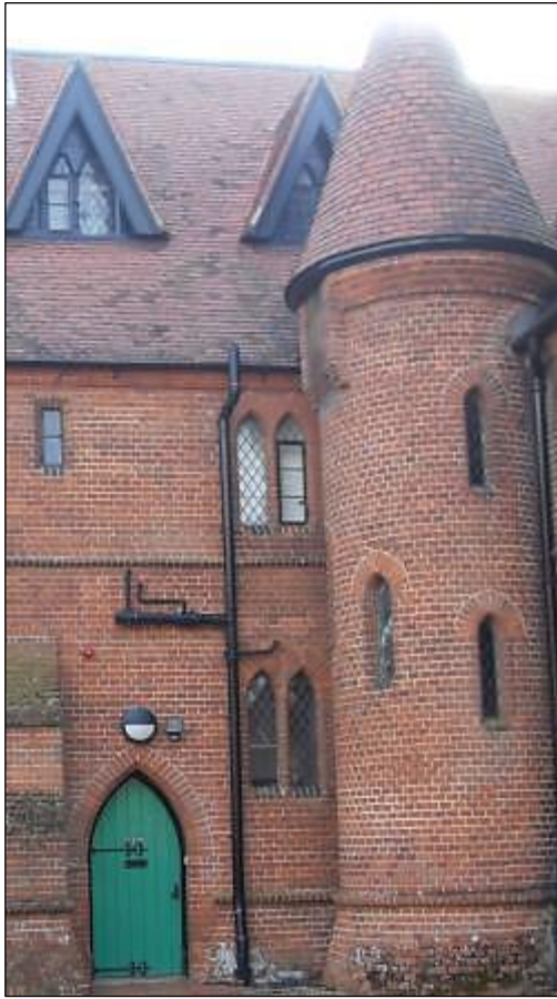
Figure 2.11 Visitors' entrance with turret housing spiral stairs to the upper room chapel, Ditchingham.
