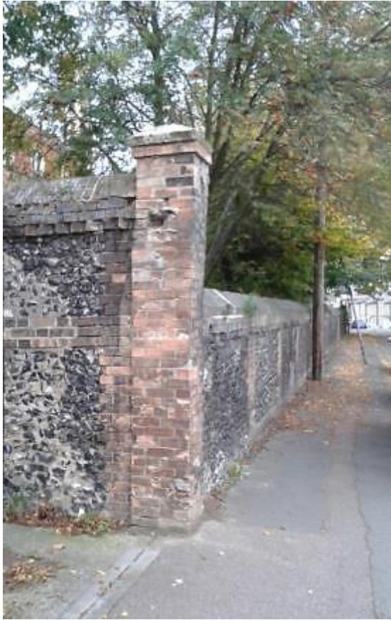
Figure 2.13 Churchyard wall abutting the Cambridge Female Refuge, twelve feet six inches high in contrast to the churchyard perimeter wall of nearer five feet.
