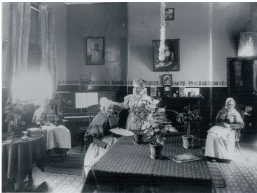
Figure 4.15 Aged Women's Day Room, Cambridge Union Workhouse, Mill Road. Frederick Leach's stencil work runs round the dado rail. No date but c.1880. Cambridgeshire Collection, Cambridge Central Library, C44.47.
