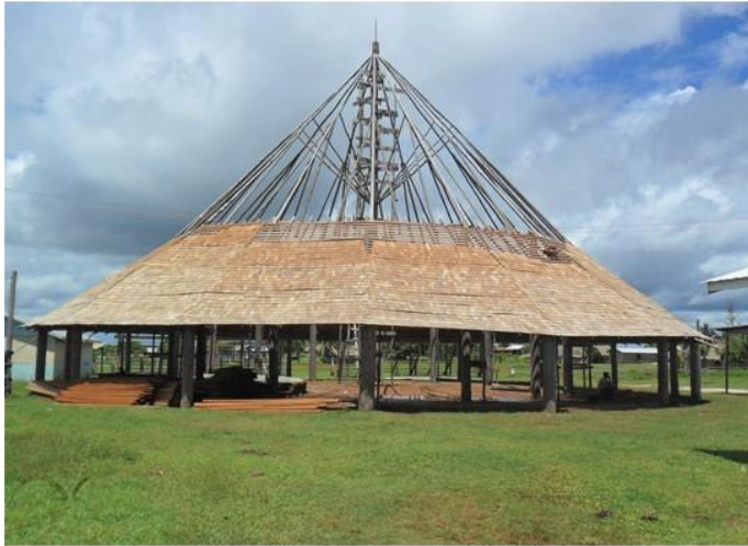
Construction of Annai benab through self help.
