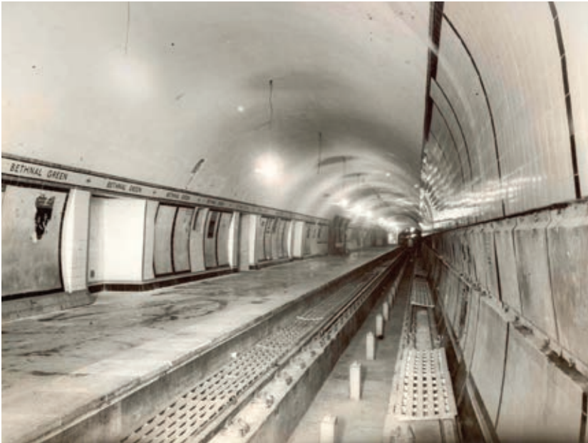
Bethnal Green station: railway under construction. Photo: Tower Hamlets Local History Library and Archives
