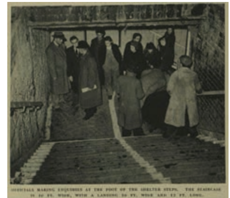
This photograph from the Illustrated London News , taken soon after the disaster, clearly shows the condition of the steps. The Dunne enquiry described them as 'plain rough concrete steps with a square wooden insertion on the edge of the tread'. It noted the concrete was 'fairly level' but the wooden edge was worn and uneven in places.
