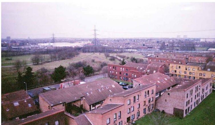
The Clays Lane complex (C. Syrett, Bishopsgate Library )
