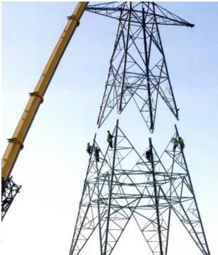
Demounting the pylons (Phil Cohen)
