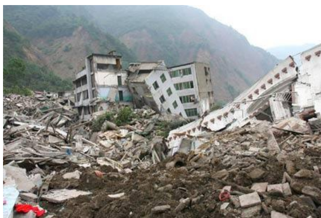
Figure 4.2 Earthquake in Sichuan, China
