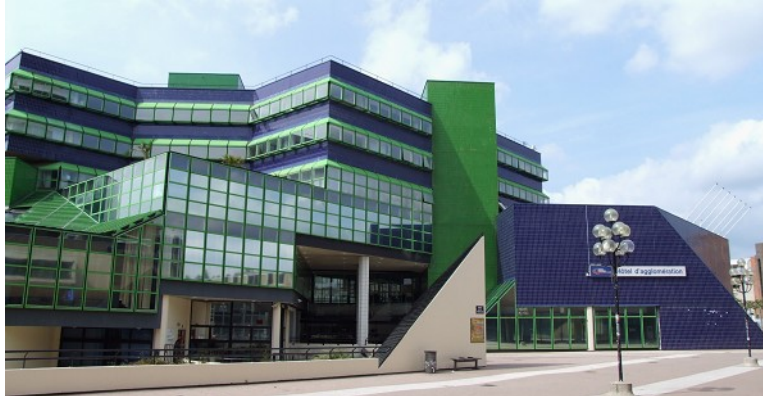
Figure 10 The cultural and administrative centre André Malraux. (Mossot, 2006)
