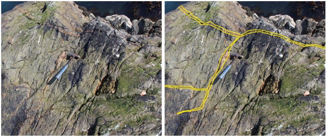
Figure 5.30: View downwards onto top surface of D44 showing sandstone wedges (yellow lines) penetrating top of D44 at Caol Ila.
