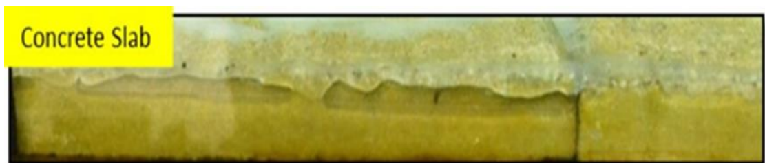
Figure 4.2: Photograph of concrete slab floor of flume tank, flow cases 1 and 2
