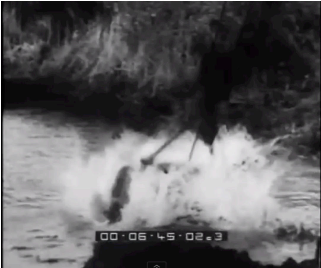
Fig. 59: The shot of the bucket that penetrates the marshy ground in the Agro-Pontine, from Dall'Acquitrino alle giornate di Littoria , 1933, Archive of the Luce Institute, Rome, consulted on 18 th November 2014.
