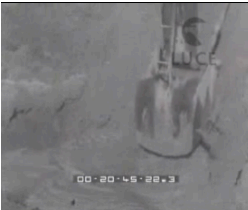
Fig. 60: The shot of the excavator while digging the marshland from: Bonifica di Piscinara , 1931, Archive of the Luce Institute, Rome, consulted on 26 th May 2014.
