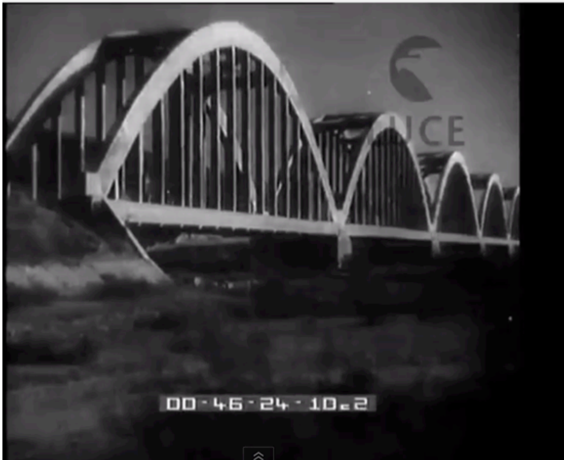
Fig. 54: A medium shot of the imposing bridge built by the Fascist regime near Durrës, from La vita della popolazione , 18 th November 1937, Archive of the Luce Institute, Rome, consulted on 13 th May 2014.
