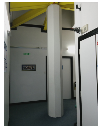
(d) The pillar which emits strong magnetic reading up to 160\mu T .
