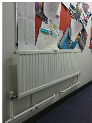
(c) The central heater which emits strong magnetic reading up to 80\mu T .
