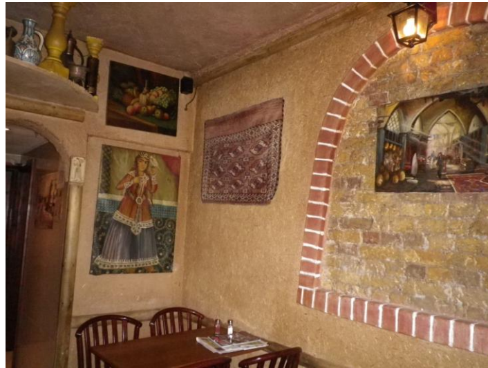
Figure 5.45 Straw and clay walls at Fanoos, Richmond, London (2012)
