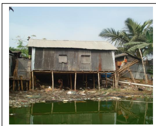
Photo 5.2: Typical housing with hanging latrine (left) in Korail. Source: Field Survey
