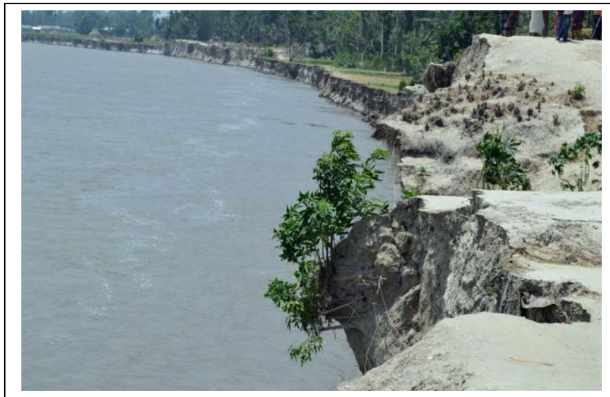
Photo 4.1: Illustrative picture of typical riverbank erosion in Bangladesh.
