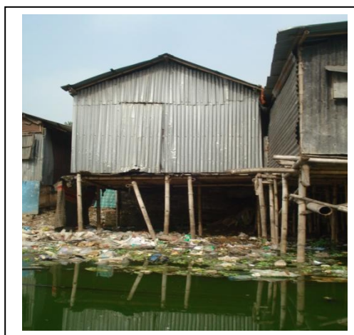
Photo 5.3: Solid waste dumping directly into the Gulshan Lake.
