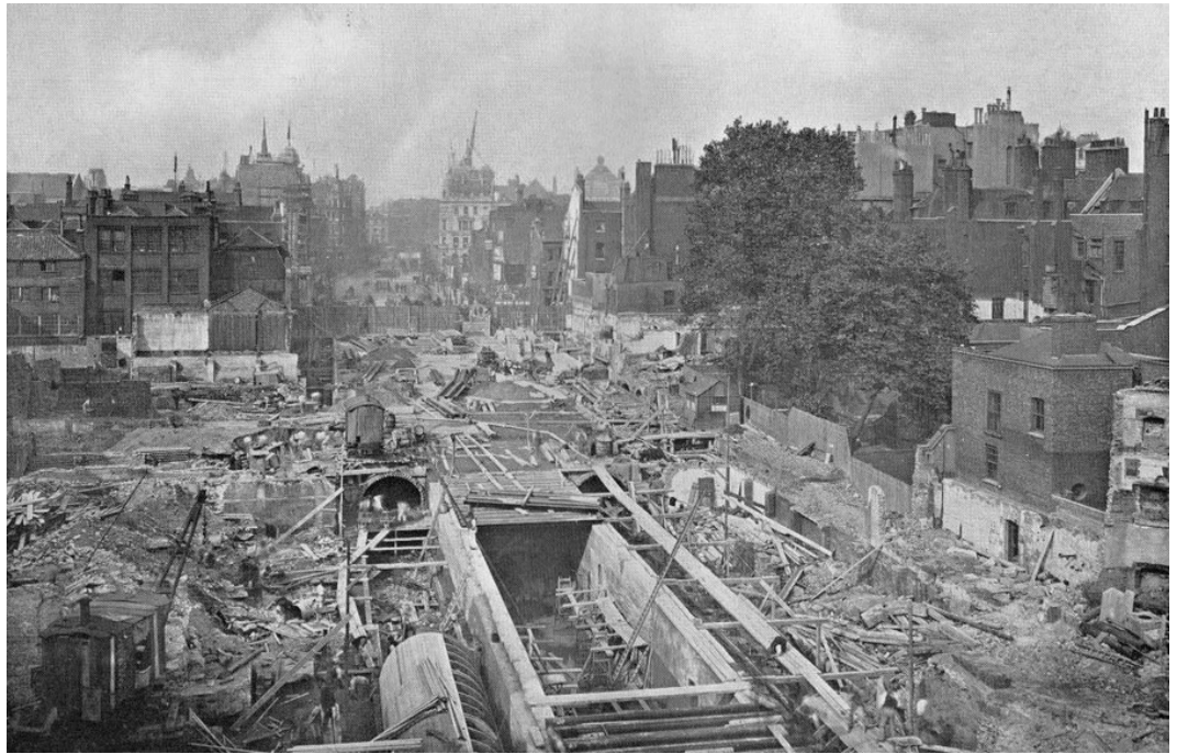
Figure 18 Kingsway Boulevard under construction, (c. 1900s) . LCC, Opening of Kingsway , p. 8.
