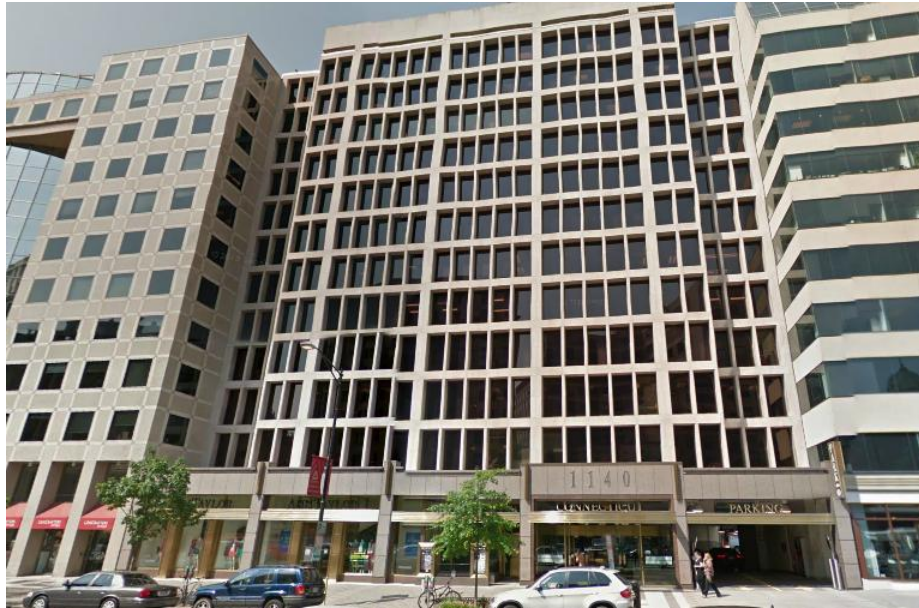
Figure 6: The headquarters of Ridge Global (Google Maps, 2013)
