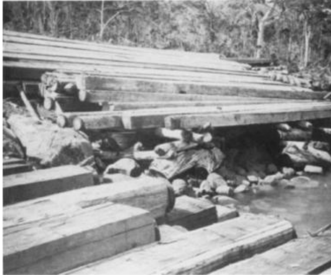
Figure 8.6 'Blue gum piles, one hundred feet long, awaiting shipment to England' 1861
