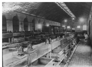
'Filtering table and boilers'
