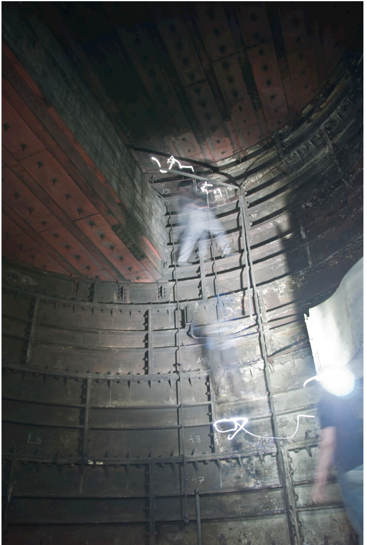
Figure 103. Gaining access to Down Street abandoned London Underground station, photo by author
