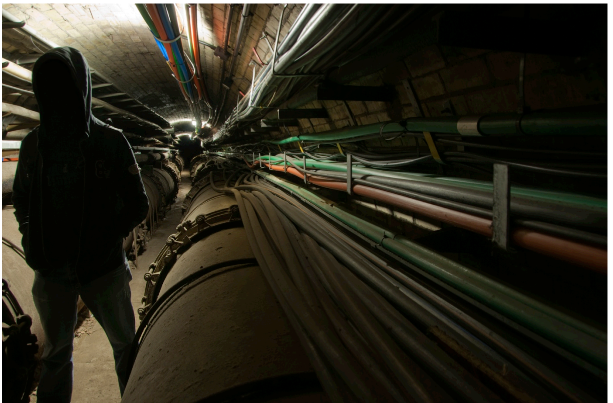
Figure 78. Marc Explo in the GLC pipe subways, one of our first live infiltrations, London, photo by author
