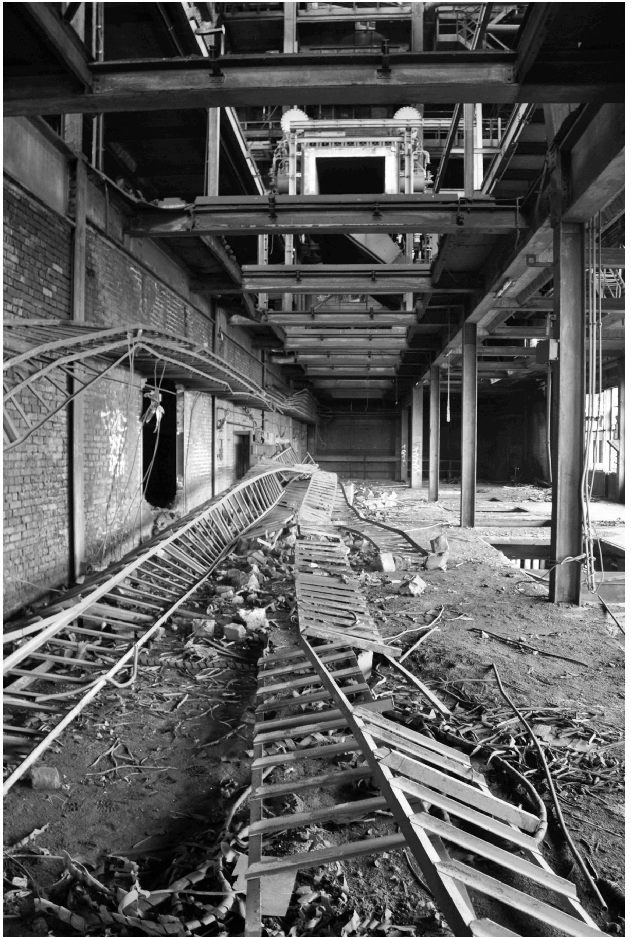
Figure 28. The abandoned factory Sinteranlage, Germany, photo by author
