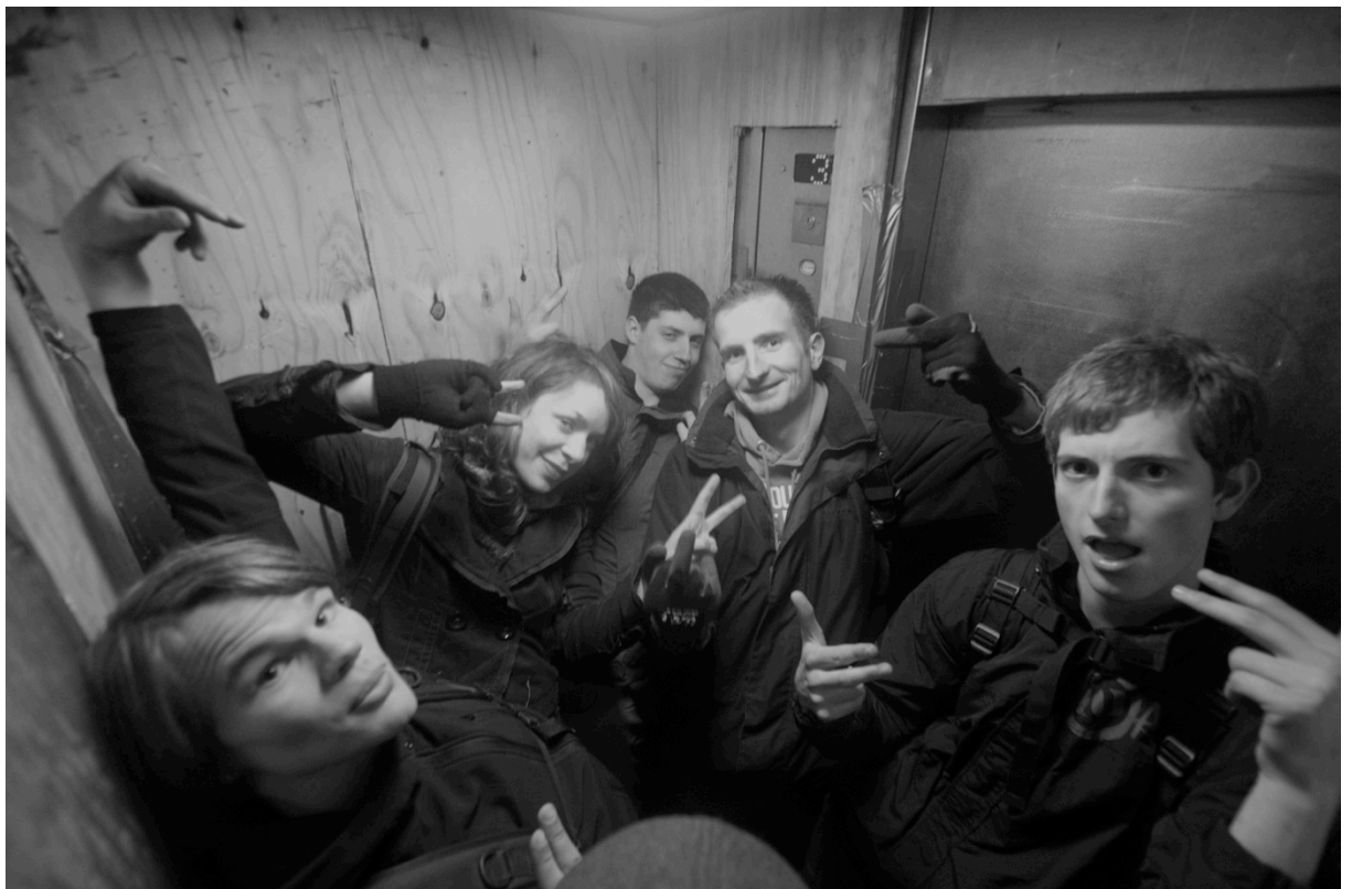
Figure 143. Activated: the LCC in King's Reach Tower, London, photo by author
