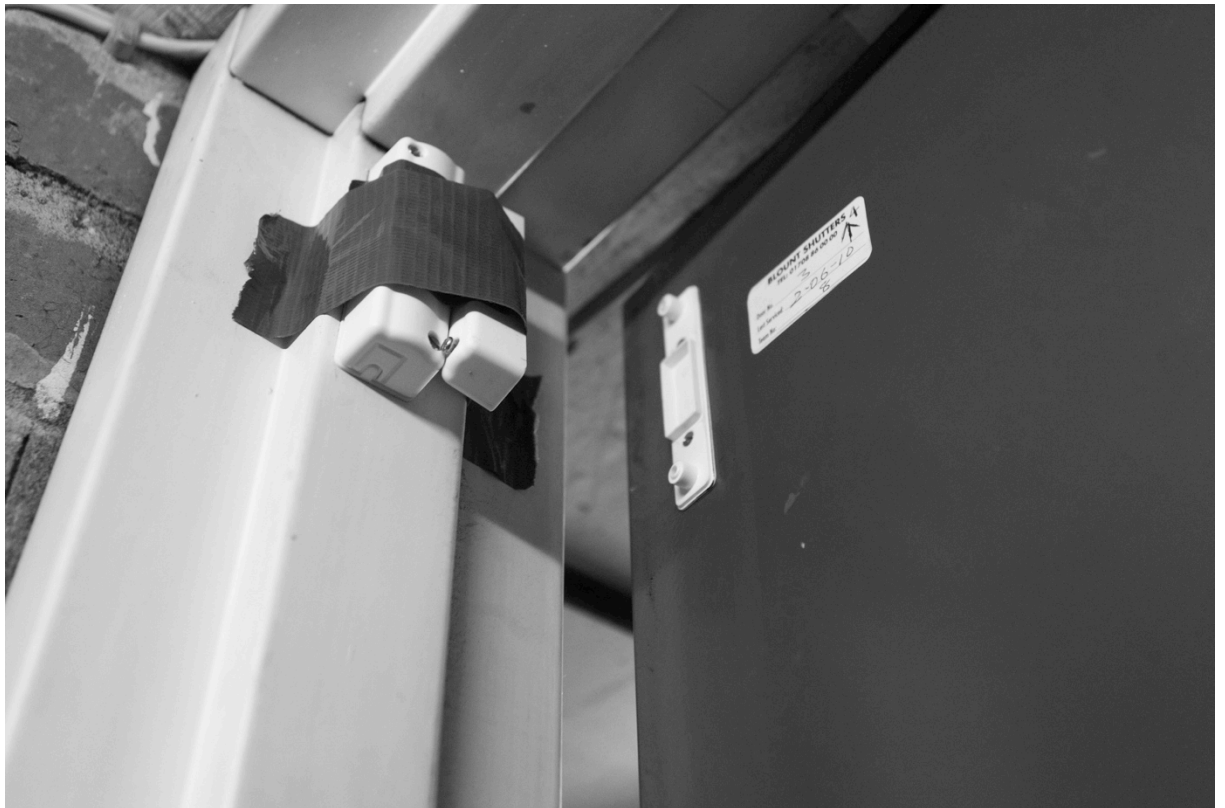
Figure 117. The disabled magnetic reed switch door alarms in the secure file storage, London, photo by Silent Motion
