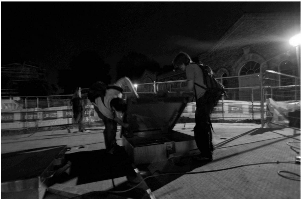
Figure 120. Security glitch located at Abbey Mills pumping station, London, photo by author
