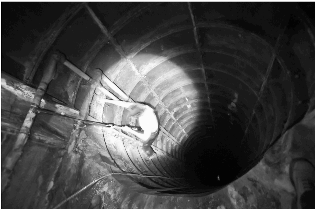
Figure 116. Silent Motion abseiling into a secure file storage through the ventilation shaft, London, photo by author
