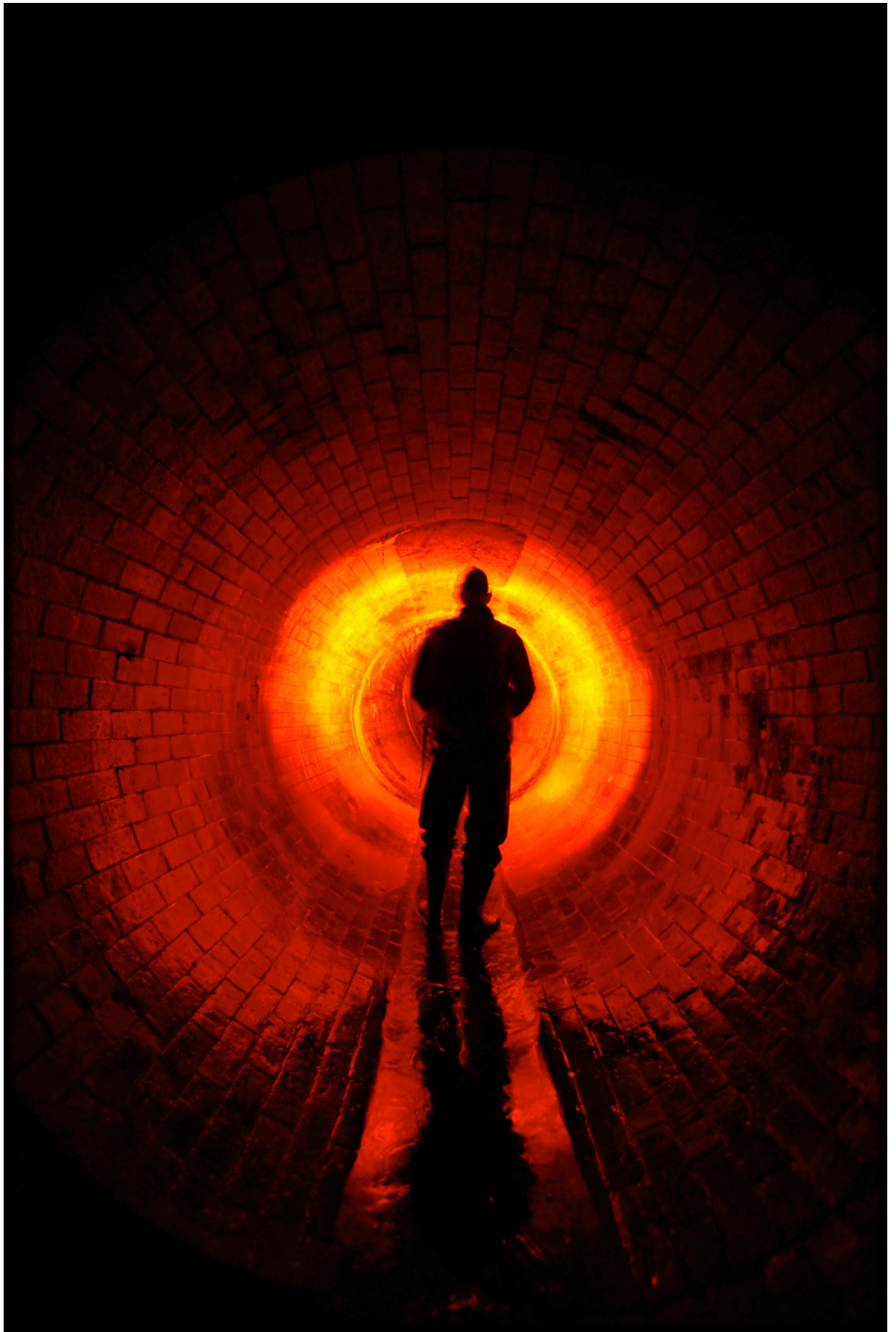
Figure 160. The author hacking Bazalgette's hidden legacy, the River Westbourne, London, photo by author
