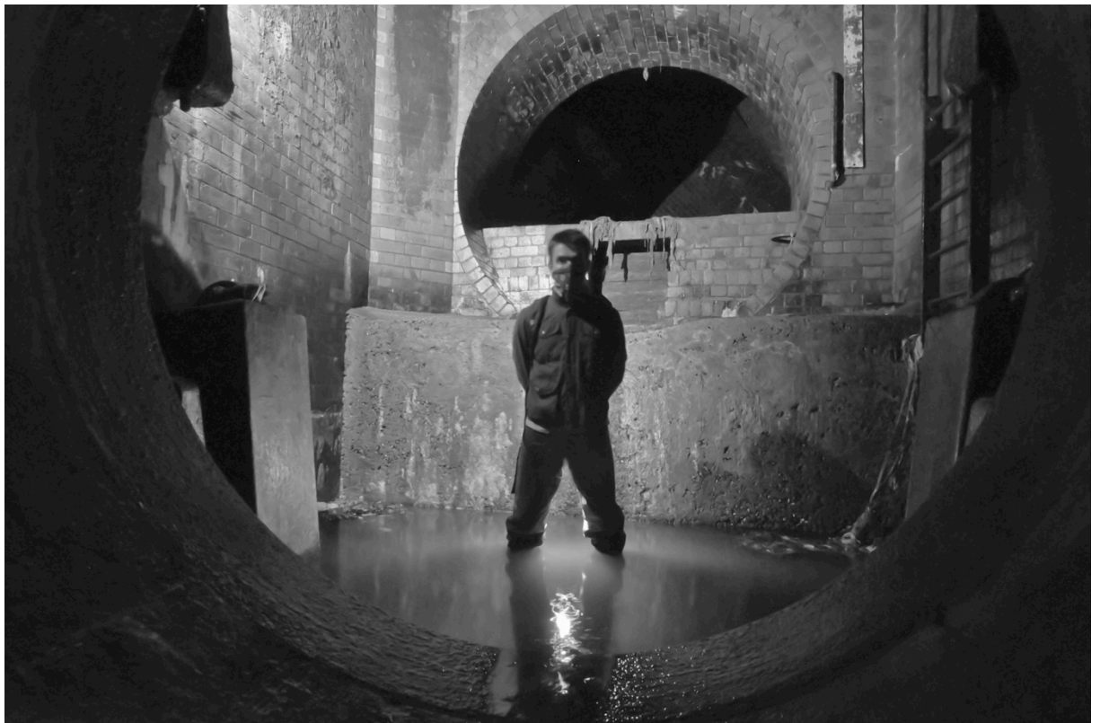
Figure 99. Author knee-deep in sewage, River Effra, South London, photo by author
