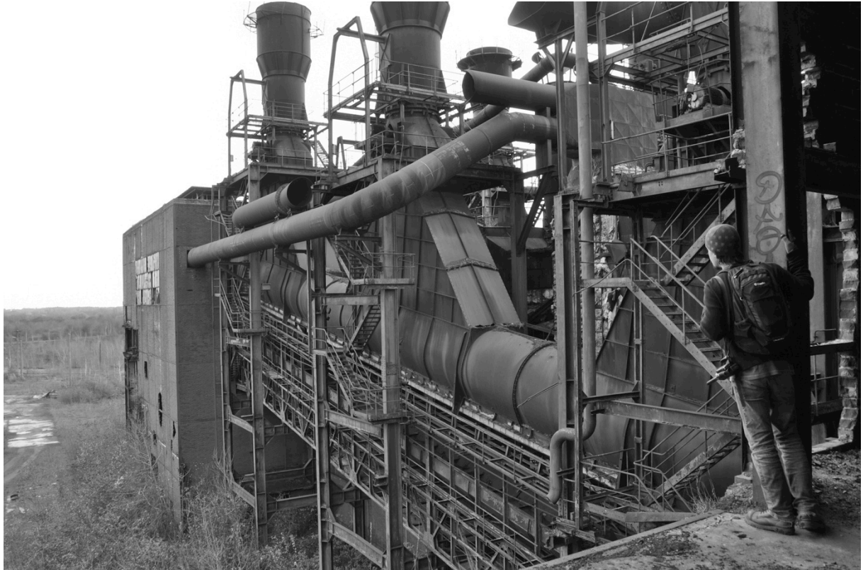
Figure 36. The author looking out over the Sinteranlage factory, Germany, photo by author
