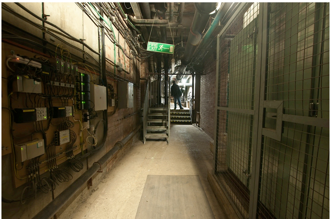
Figure 86. Patch in the Barbican utility tunnels, London, photo by author
